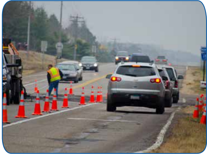
Fines for speeding through a work zone were increased in 2014.
